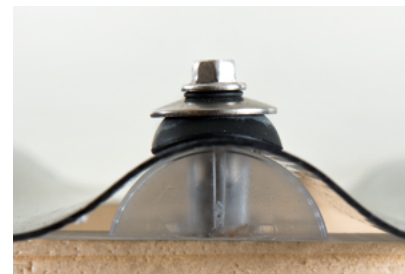
Fixing detail
